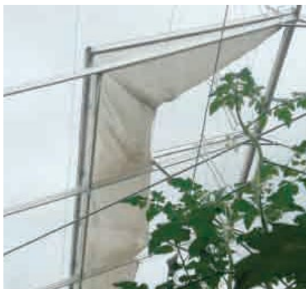
Insect-proof screen in roof opening.
